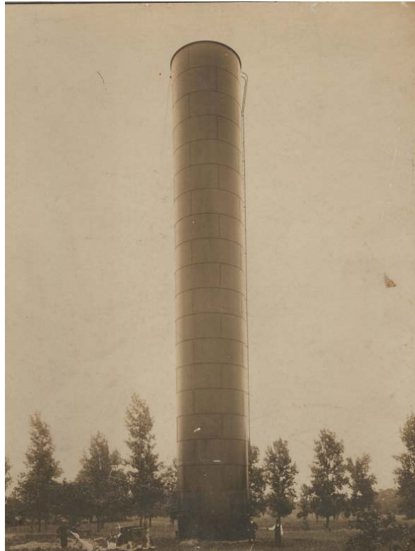
Wenonah's 100-foot high standpipe.
